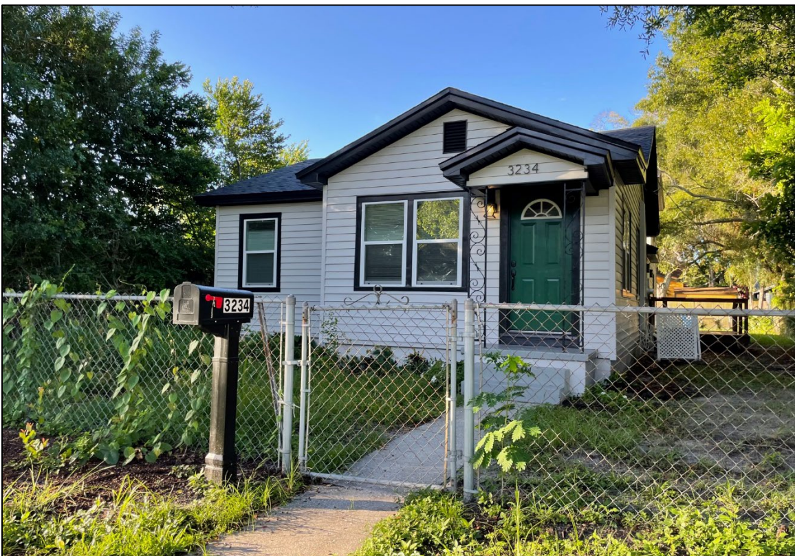
Figure 7: Photograph showing the already installed fanlight style door. The windows shown in the photograph are proposed to be replaced.
