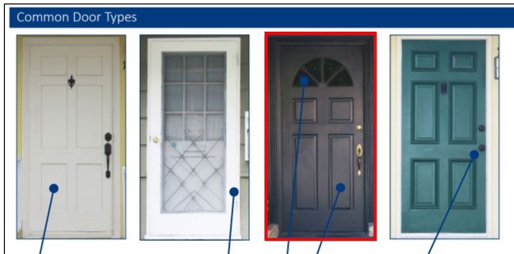
Figure 5: Common door types from the City of Anaheim's "Architectural Style Guide: Minimal Traditional." Fanlight door outlined in red.
