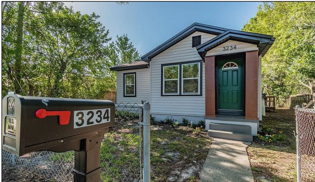
Figure 3: Photograph depicting the unapproved work.
